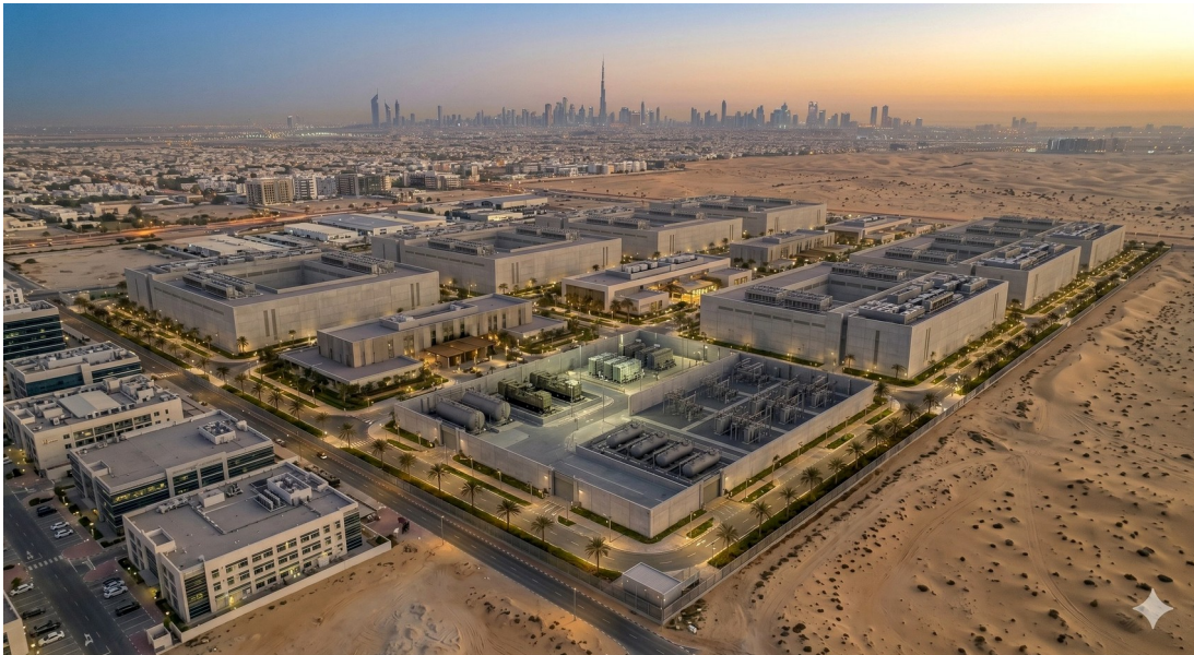
Editorial visual: large-scale digital infrastructure in the Dubai environment. Image credit: VOLT Datacenters.
